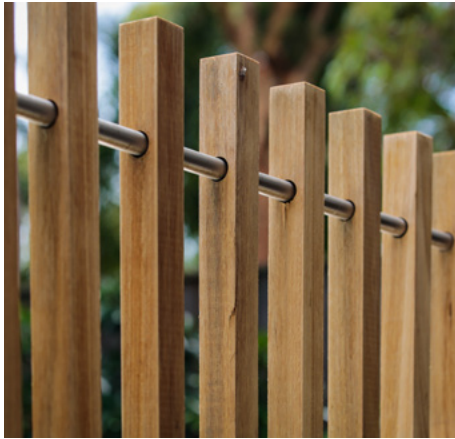
Front Fence Type B & owner installed secondary fencing for corner lots only.
