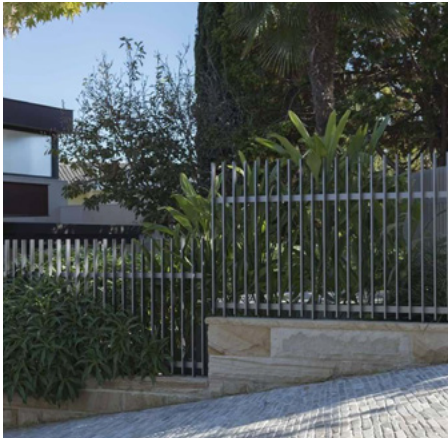
Front Fence Type C & owner installed secondary fencing for corner lots only.
