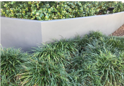
RENDERED AND PAINTED BLOCKWORK
