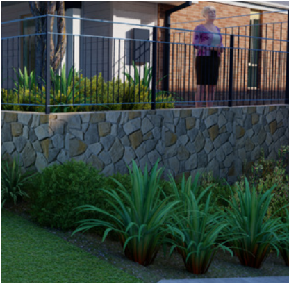
Rendered Masonry – Stone Clad
