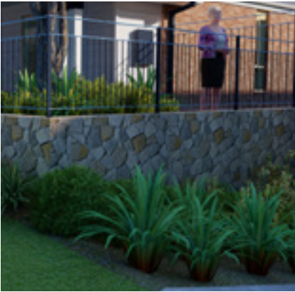
Rendered Masonry – Stone Clad
