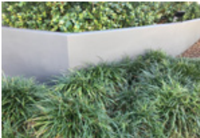
RENDERED AND PAINTED BLOCKWORK
